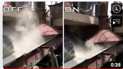
Yansons Effective Dust Extraction System at Primary Crusher
