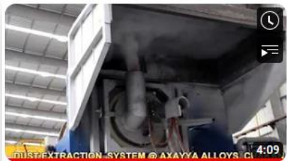
Yansons Engineering Air Pollution Control Equipment Installations 2019
